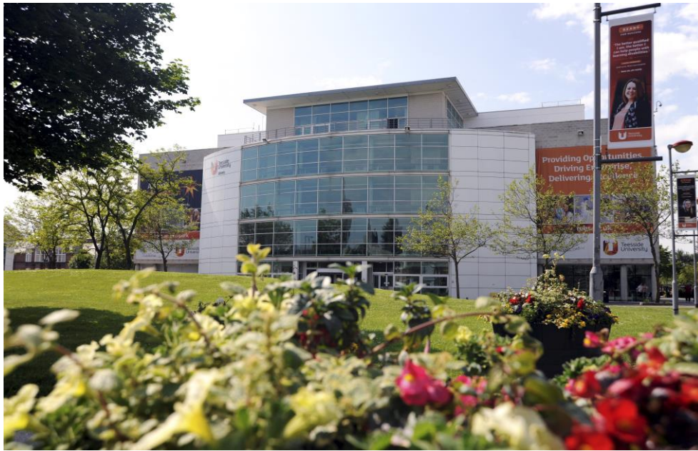
Figure 1: Front of the library, showing no natural light at the corners of the building
